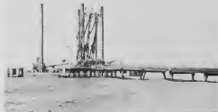
The GEM-111, a self-elevating work barge, arrived December 15 and docked at Lago's Sea Berth where it will be engaged in improving the offshore berth.
